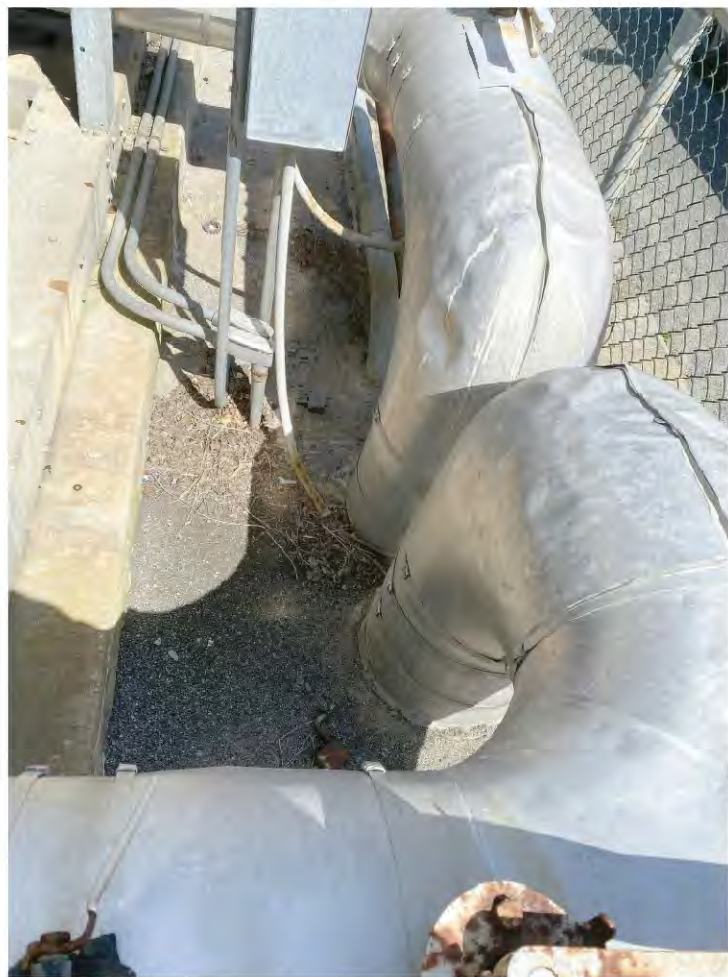
C CHILLED WATER PIPING TO BELOW GRADE SCALE: NTS
